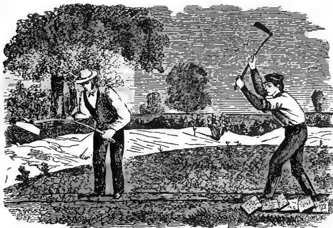
Fig. 10.—CUTTING AND PARING TURF.
